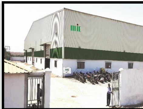
Pune - Alandi 10,000 MTPA
