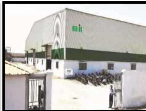
Pune - Alandi 10,000 MTPA
