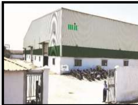
Pune - Alandi 10,000 MTPA
