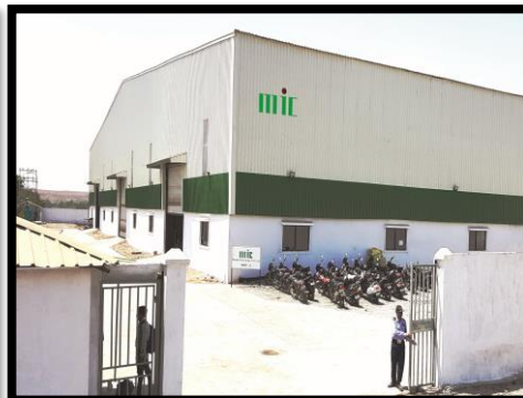
Pune - Alandi 10,000 MTPA
